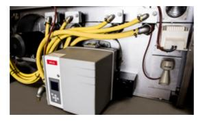
Easy maintenance Can be built-in on three sides and ergonomically designed: All key service units can be accessed quickly and easily from the front
